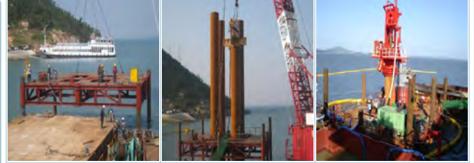
Erecting Jigiaket Driving sacrificial steel pipes Conducting offshore RCD excavation
